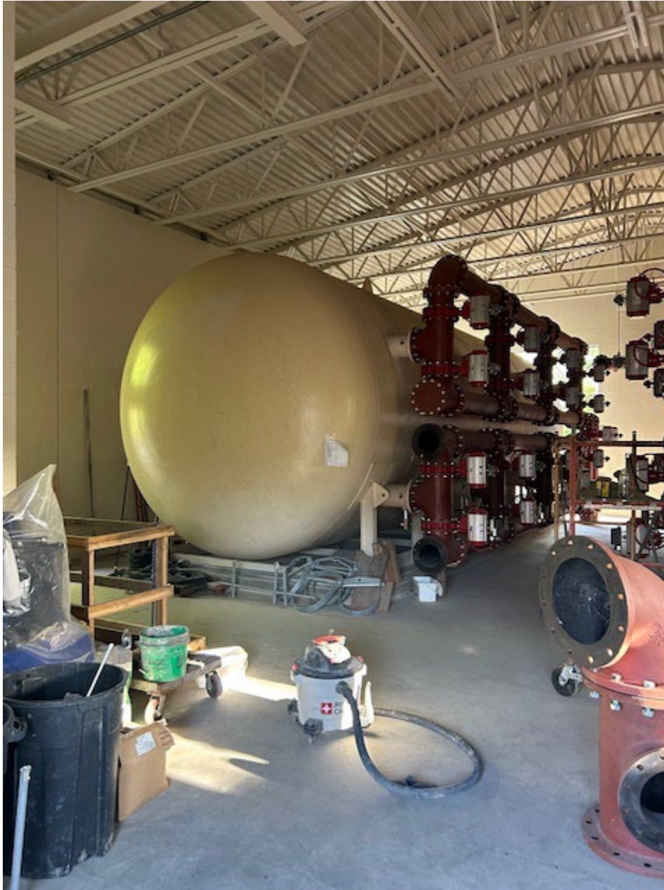
One of the two pressure vessels in the facility
