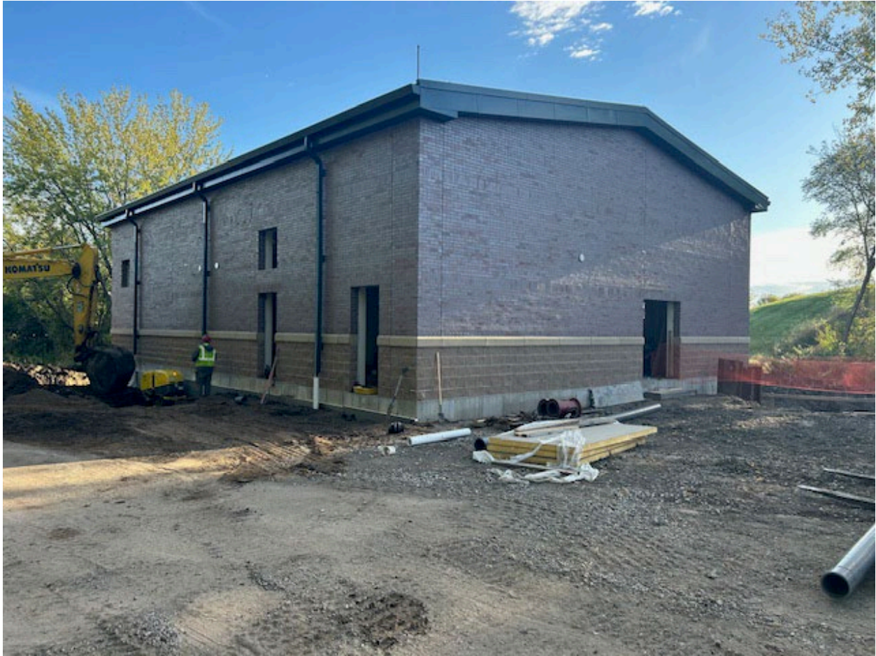
Exterior Masonry and roof installed
